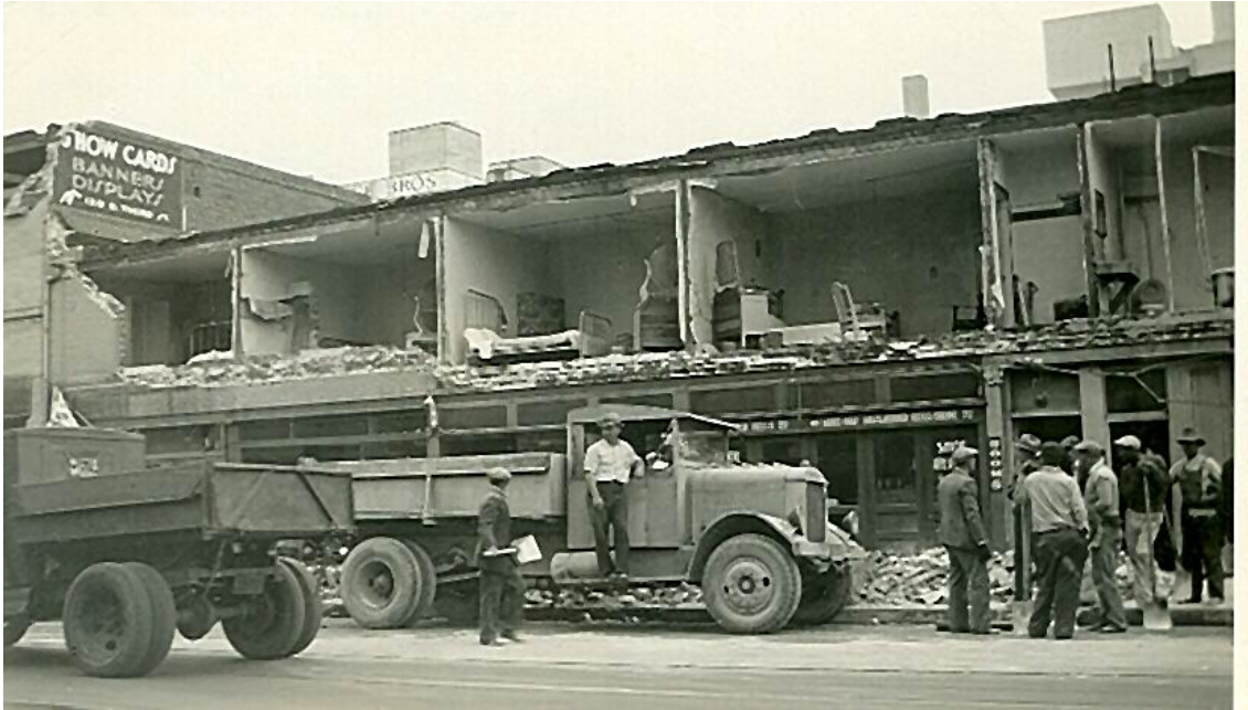
Damage caused by March 10, 1933, Long Beach Earthquake (photo by M. Biot)
